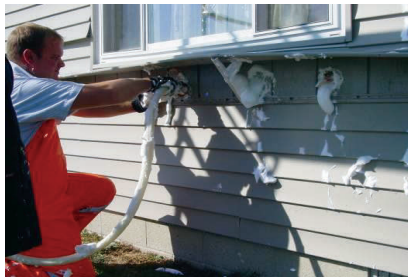
Figure 214-4-1: Injection foam being used to insulate wood frame wall
