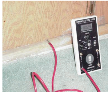
Figure 114-1-1: Toe-kick sealed with duct mask tape; pressure pan reading of 24 Pa!
