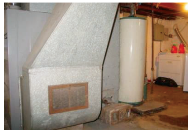
Figure 315-3-1-6: Return air grilles should be sealed
