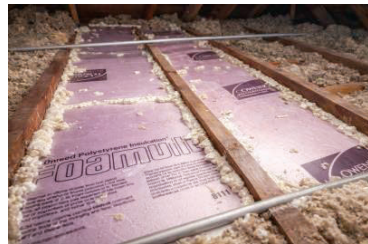
Figure 212-2-2: Soffit sealed with foam board and 2-part spray foam
