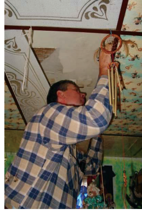
Figure 111-1-2: Remove a ceiling tile to relieve
