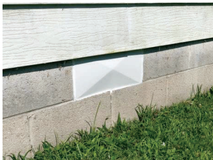
Figure 215-5-1: Insulated vent with metal cover.
