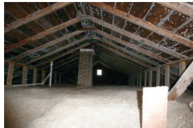
Figure 212-2-8: Cut-off chimney in attic
