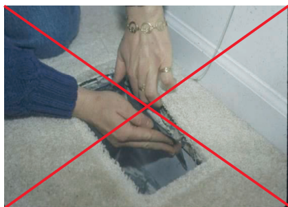
Figure 315-3-2-1: Tape is not to be used for sealing ducts in the Illinois WX Program
