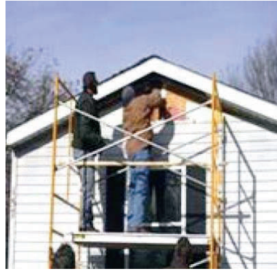
Figure 416-3: Insulating a post-HUD mobile home from the gable end. Courtesy US Dept. of Energy
