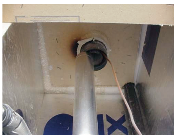
Figure 311-1-1-3: Ensure that vent is properly connected
