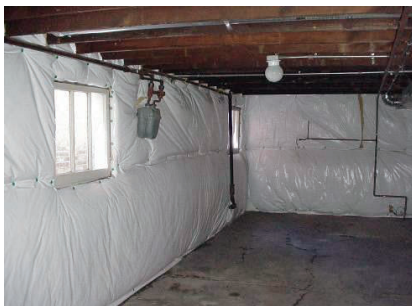
Figure 216-2-1: Vinyl faced fiberglass insulation
