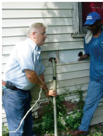
Figure 214-2-1: Dense-pack cellulose being installed
