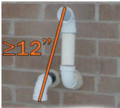
Figure 314-1 Goose neck venting
