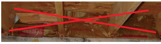
Figure 217-1: Batt insulation is not permitted to be used for box sill insulation
