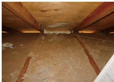
Figure 212-2-13: Exterior wall top plate under low-pitch roof sealed with foam.
