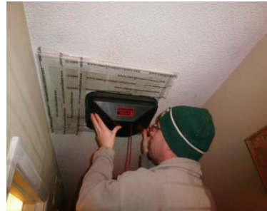
Figure 114-1-2: Duct partially covered with duct mask tape.
