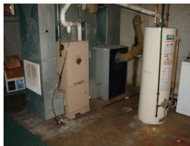
Figure 312-2: Combustion appliance zone: note presence of grille in return air duct that can cause depressurization of the water heater
