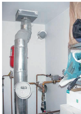
Figure 312-4-2: Combustion air intake
