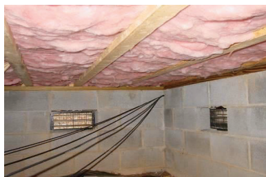
Figure 215-2-1: Insulation should fill floor cavity
