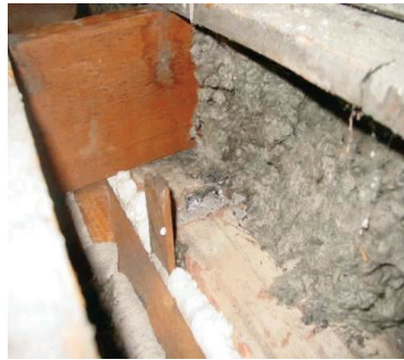
Figure 212-2-6: Fur cavity sealed with 2-part spray foam
