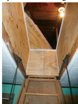
Figure 213-5-2: Box around retractable attic stairs
