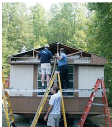
Figure 416-2: Insulating an older single wide from the gable end. Courtesy US Dept. of Energy
