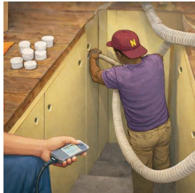
Figure 213-5-3: Stairwell walls being dense-packed
