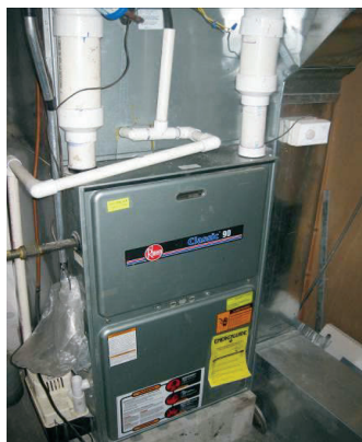
Figure 313-3-1: Direct vent sealed combustion furnace
