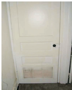
Figure 312-4-3: Transfer grille
