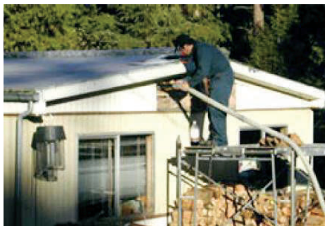
Figure 416-1: Insulating an older double-wide from the gable end. Courtesy US Dept. of Energy
