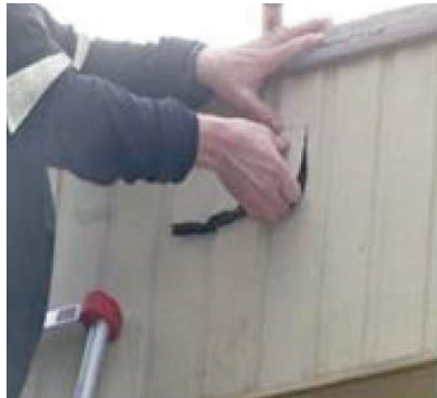
Figure 416-4: Accessing the attic cavity in a mobile home. Courtesy US Dept. of Energy
