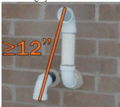
Figure 319-2-2 Goose neck venting
