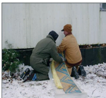
Figure 415-2-1-1: Batt-stuffing a mobile home wall
