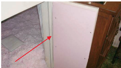
Figure 213-6-5-1: Knee wall hatch insulated and weatherstripped
