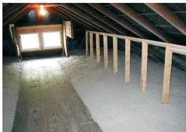
Figure 213-3-2-1: Insulation blown under floor boards and then over floor boards where client storage is not needed
