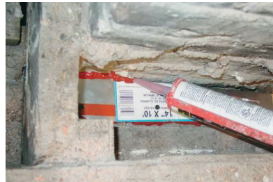
Figure 212-2-7: Seal chimney bypass with sheet metal and high temperature RED sealant
