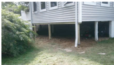
Figure 215-4-1: Crawl space supported on piers
