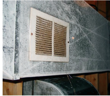
Figure 315-3-1-4: Permanently seal registers in unconditioned
