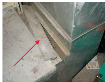
Figure 315-3-1-2: Metal filter
