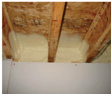
Figure 217-1-1: Two-part spray foam on box sill
