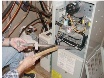
Figure 311-1-1-2: Clean burners with stiff brush
