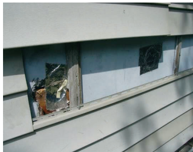
Figure 214-2-2: Hole sealed with sheathing tape
