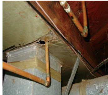
Figure 315-3-1-5: Seal holes in ducts
