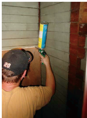
Figure 212-4-2-1: 1-part spray foam; foam canister is screwed onto a foam gun
