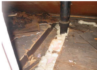
Figure 212-2-9: Plumbing wall cavity sealed with foam board and 2-part spray foam
