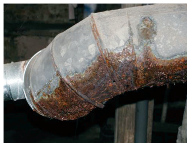
Figure 311-1-1-4: Check vent for condensation problems
