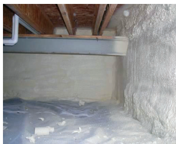
Figure 215-1-2: Two-part spray foam applied to foundation wall with ground cover
