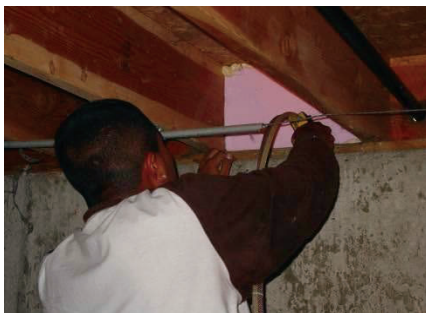
Figure 217-2-1: Rigid foam board sealed in place with 2-part spray foam
