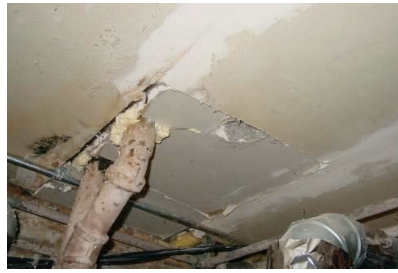
Figure 212-2-11: Cavity beneath bathtub sealed with gypsum board and dense-packed with cellulose
