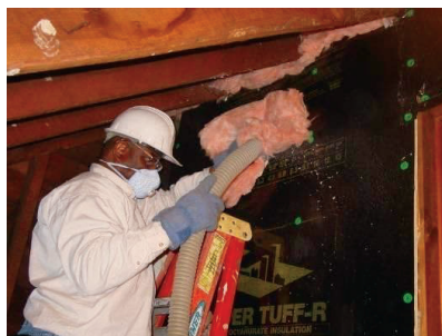
Figure 213-6-4-3: Knee walls being dense-packed with cellulose
