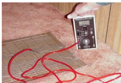
Figure 411-4-4-1: Initial pressure pan reading of 47 Pa; return duct was totally disconnected
