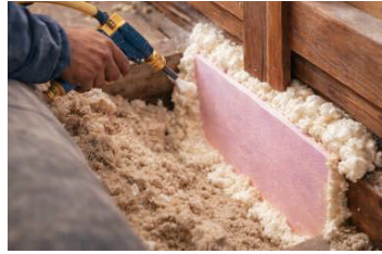
Figure 212-2-1: Sealing joist cavity under knee wall with foam board and 2-part spray foam
