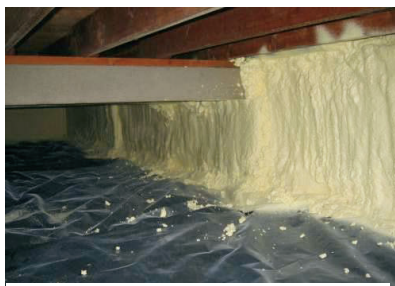
Figure 215-4-2: Minimum 6 mil ground cover; sealed to foundation wall with 2-part foam
