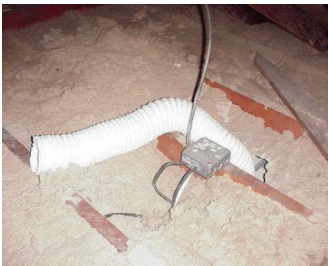
Figure 507-1: Fans may not be vented into the attic under the Weatherization Program
