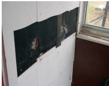
Figure 214-1-1: Asbestos siding that has been removed
