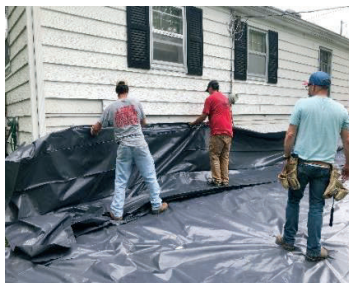
Figure 513-6-3: Exterior Containment
