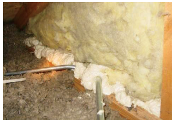
Figure 212-2-3: Stud cavity sealed with 2-part spray foam
