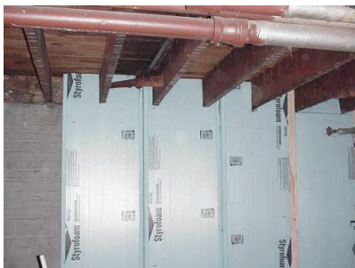
Figure 216-1-1: Rigid foam board basement wall insulation
