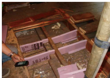
Figure 213-1-5: Rigid foam board used as barrier next to K&T wiring; floor cavity will be blown with cellulose insulation
