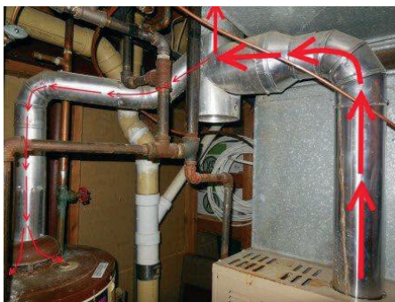
Figure 312-3: Checking for spillage at the water heater after firing the furnace
