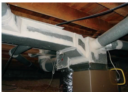
Figure 315-3-2-2: Duct mastic used to seal duct joints
