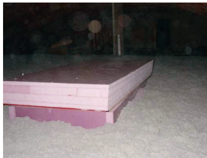
Figure 213-5-1: Attic hatch insulated with foam board; plywood blocking has been insulated with foam board
