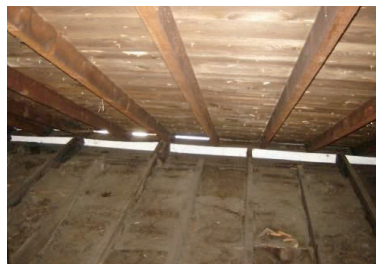
Figure 213-2-4-1: Foam blocking installed over top plates
