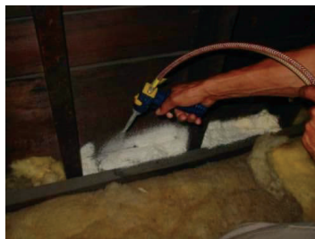
Figure 212-2-4: Study cavity blocked with batt insulation and sealed with 2-part spray foam
